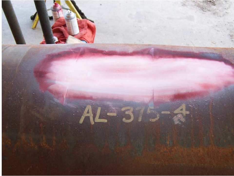
Figure 3 - Dye penetrant used to ensure gouge removal by grinding
