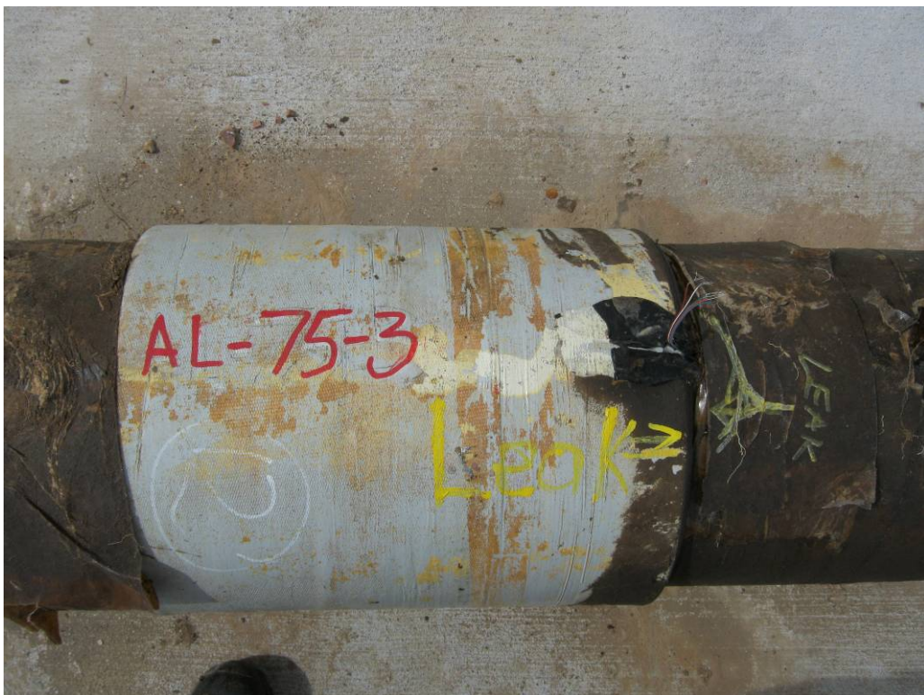
Figure 6 – Photograph of Failure Location, 75% Corrosion Sample
