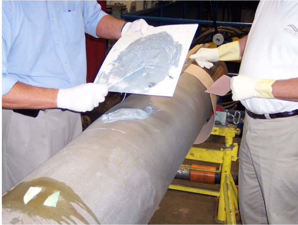
Figure 5 - Epoxy material used to fill the dented region
