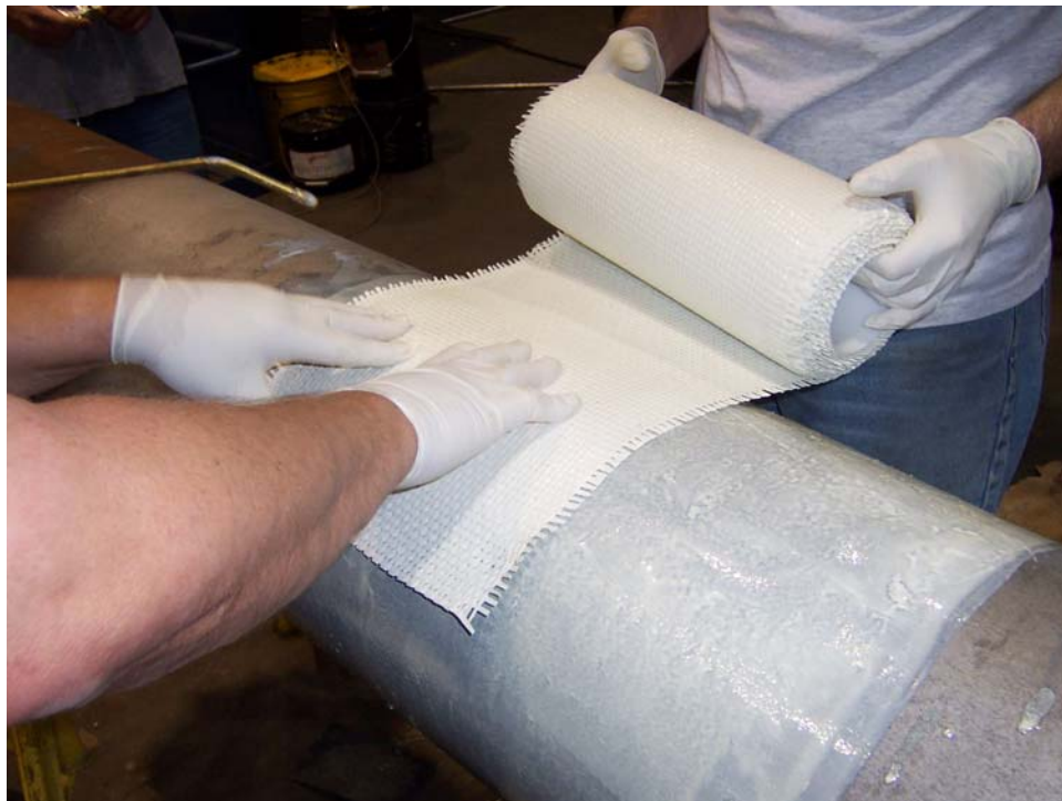
Figure 6 - First layer of Aquawrap™ installed on pipe
