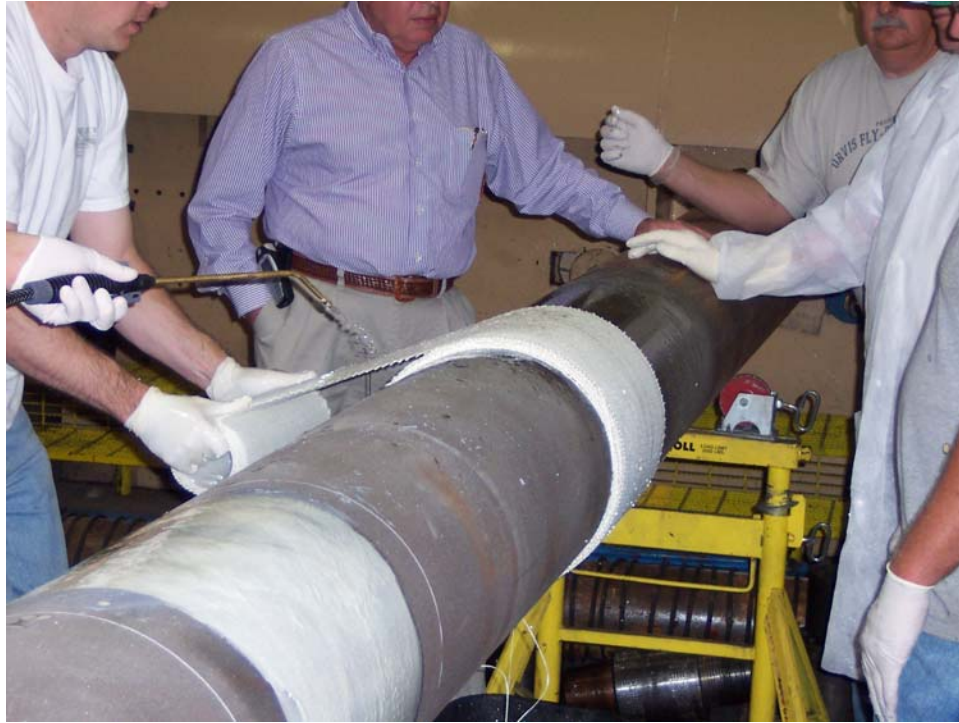
Figure 7 - Continued wrapping of Aquawrap™ in repairing damage
