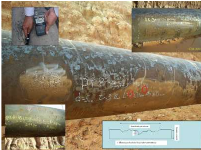
External corrosion direct assessment (ECDA)
