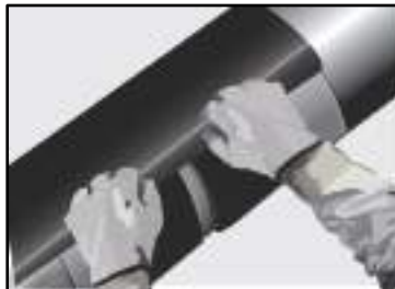
Figure 8: Positioning the sleeve
